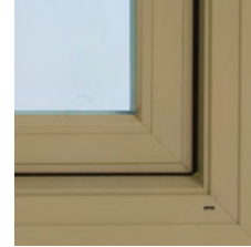
Clad Brickmould Corner
