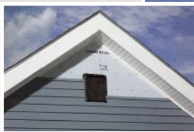
Gable Vent Base installed with siding
