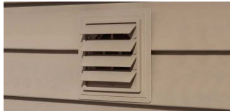
Louvered Exhaust Vent Louvered Exhaust Vent is used to vent dryers and bathroom exhaust fans.
